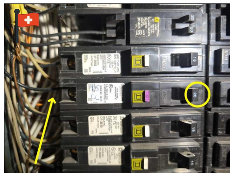
Circuit breaker #15 - 20 amp breaker with 14 AWG branch circuit wiring connected. A 20 amp breaker requires a minimum 12AWG copper wire. This is an unsafe configuration that should be corrected by a qualified electrician.
