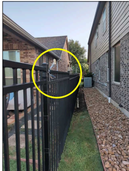
Perspective photo of the irrigation system's rain/moisture sensor.
