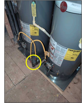
Perspective photo showing the gas shutoff valves for the water heaters.
