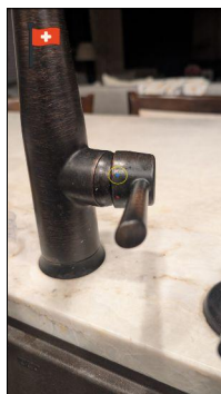
Kitchen faucet handle in down position - cold water should flow (hot flows instead).
