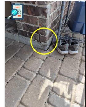
Example of a corner pop on the south-central corner of the homes foundation where repair is recommended.
