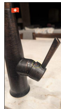
Kitchen faucet handle in up position - hot water should flow (cold flows instead).
