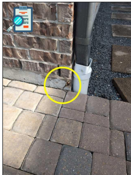
Example of a corner pop on the southeast corner of the homes foundation where repair is recommended.
