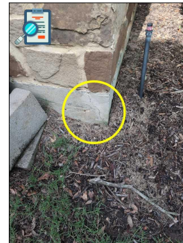
Example of a corner pop on the northeast of the homes foundation where repair is recommended.
