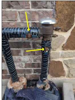
Perspective photo of the irrigation water shut off valve.
