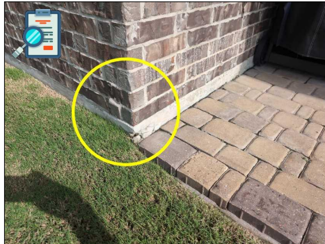
Example of a corner pop on the south-central area of the homes foundation where repair is recommended.
