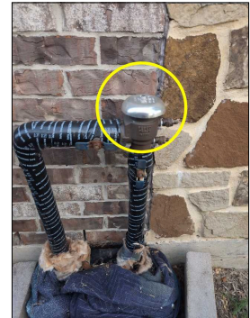
Perspective photo of the backflow prevention device.
