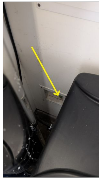
Main water shutoff in garage behind water softener system.
