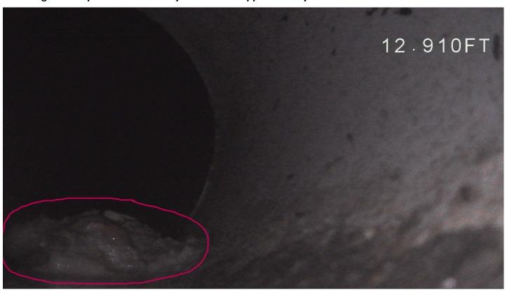
**Sludge buildup – approximately 16ft.** (This is just one example. In the videos there are several locations where this type of buildup is visible.)
